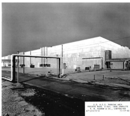
Figure 11. C-331 Process Building Completed
