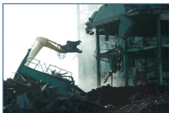
Figure 19. Demolition of C-340 Structures
