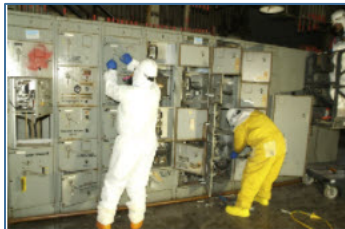
Figure 18. Workers deactivate C-340 Instrument Systems
