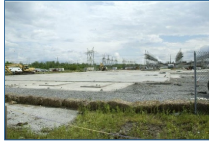
Figure 20. The C-340 Site following Demolition
