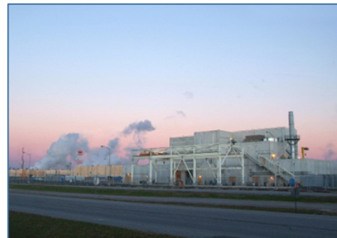
Figure 15. The PGDP DUF_6 Conversion Facility
